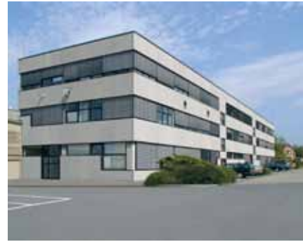
Carrier Lead Design Center in Deutschland
